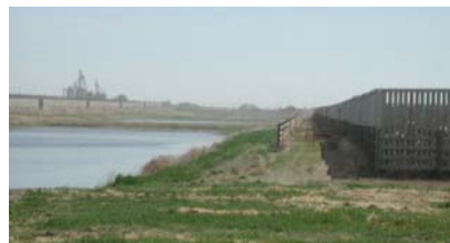
Figure 17 Back alley and containment cell
